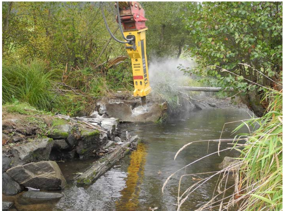
Figure 17: The removal of one of the last remaining barriers in the Mitternacher Ohe. (© Landesfischereiverband Bayern e.V.)
